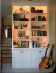
**Built-in Book Shelf.** All frame and panel construction, hidden rope lighting in routed groove behind shelf unit face frame.
